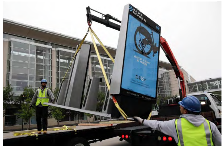
Figure 2.5: Bike Share Station Lifted into Place in Chicago.
